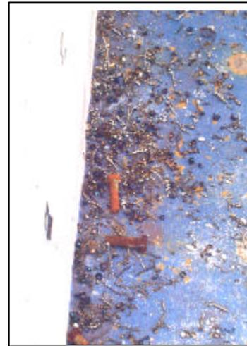
**Figure 3. Metal shavings on walking surface after cutting completed.**
