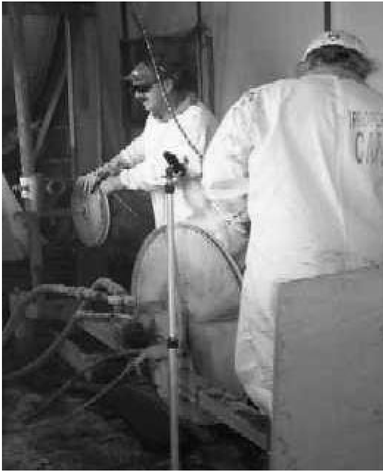
Figure 4. The diamond wire system (hydraulic power unit is outside containment).
