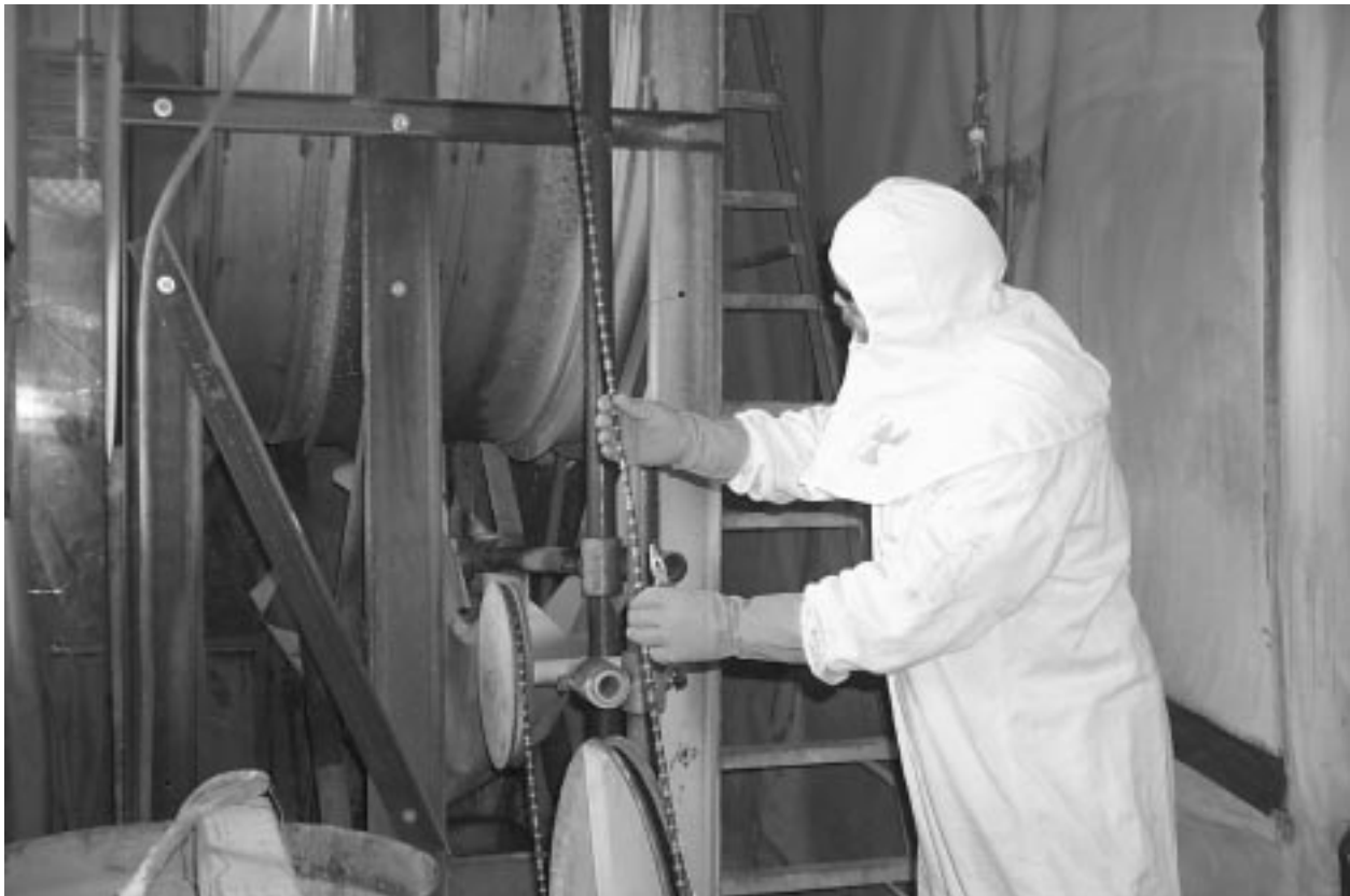
Figure 3 Diamond Wire Rope and Pulleys
