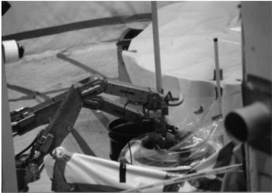
Figure 2. The DAWP size reducing and packaging a highly activated reactor component.
