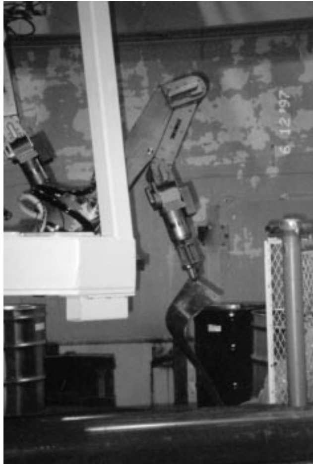
Figure 5. The DAWP Removes Material from the Reactor Top for Disposal
