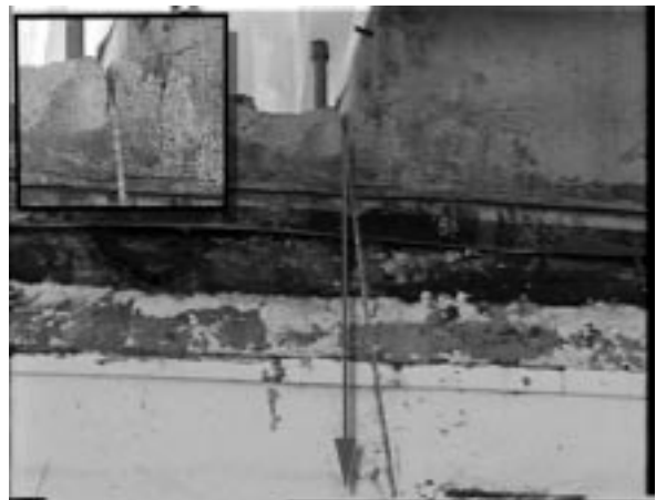
Figure 1. Diamond wire and cut line.
