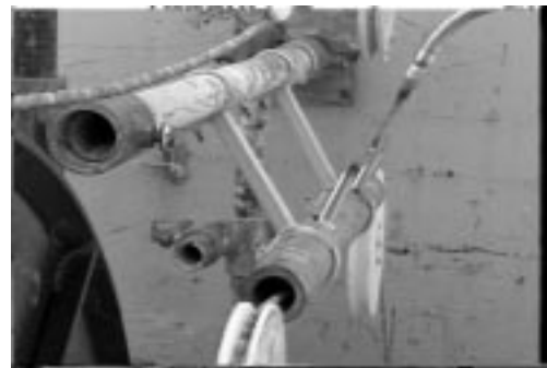
Figure 5. Cooling pipe housing for applying liquid nitrogen to the diamond wire.
