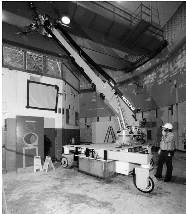
Figure 1. Rosie at CP-5, boom extended with jackhammer end-effector.
