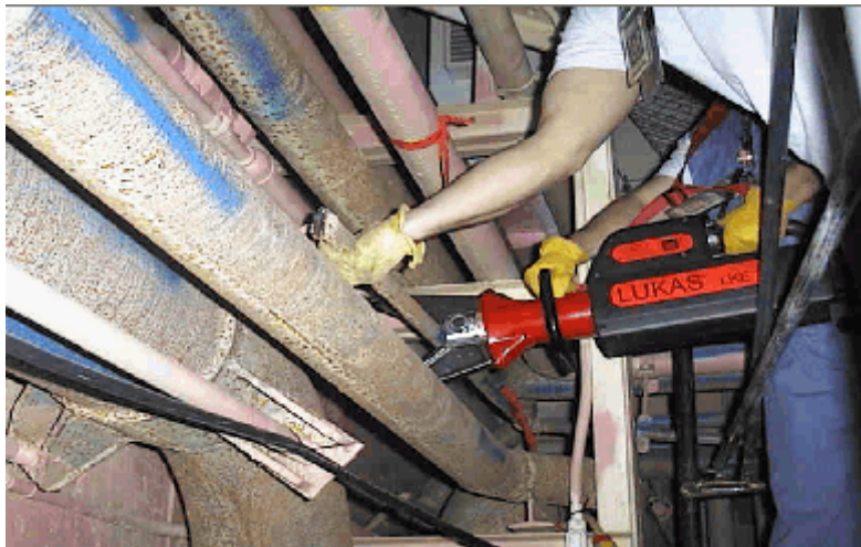
Figure 3. Typical cutting with the innovative shear.
