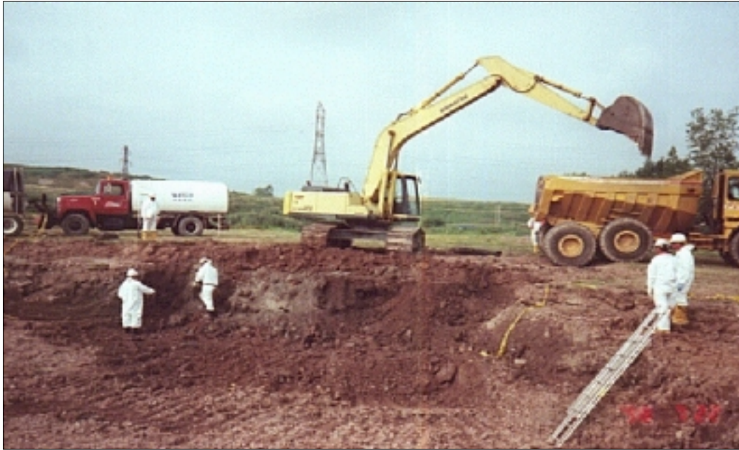
Figure 7. ASAP mode used for precise excavation of soils.
