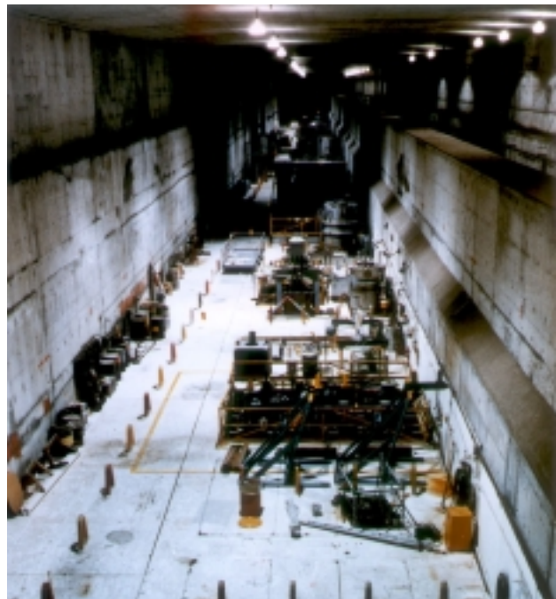
Figure 5 221-U facility (canyon) deck.
