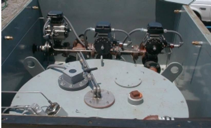
**Figure 6. Waste Stream Consolidation System – surge tank top view, inside secondary containment.**
