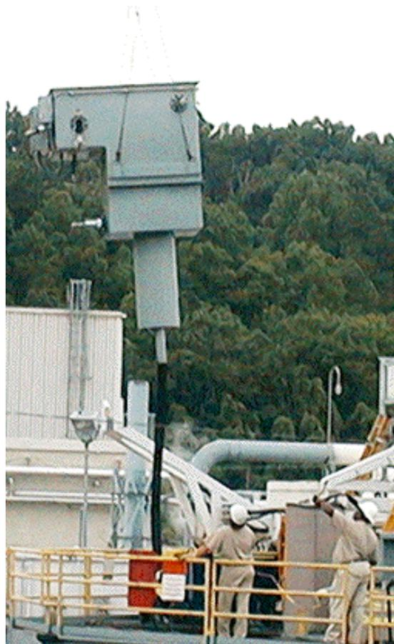
**Figure 5. Waste Stream Consolidation System – surge tank during installation at Gunite and Associated Tanks Operable Unit, Tank W-9.**
