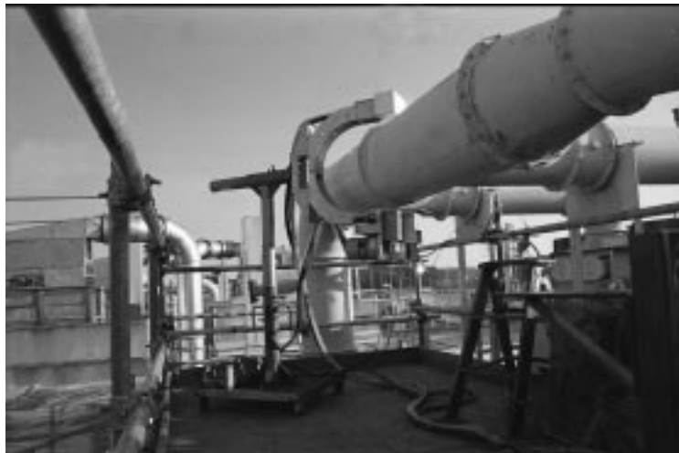
Figure 1. Inspection Head on 20-Inch Diameter Ventilation Duct
