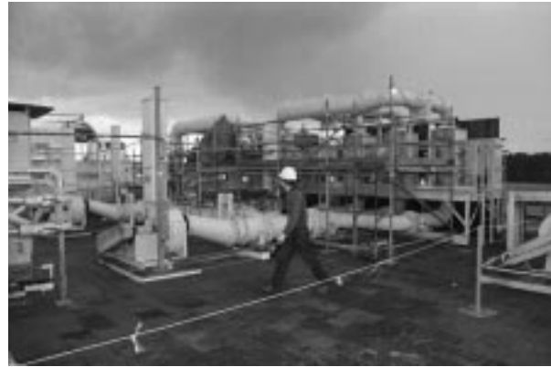
Figure 4. Exhaust System with Scaffolding
