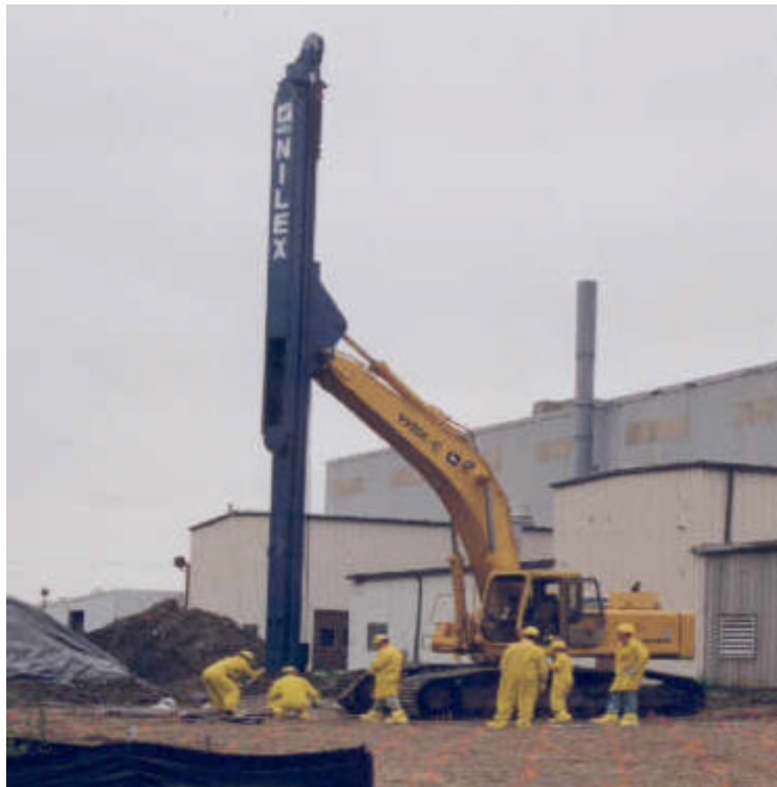
Figure 4. PVW mandrel installation system.
