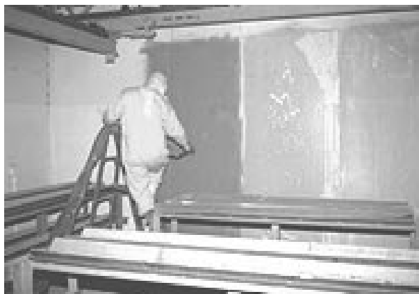
Figure 3. Application of ALARA™ 1146 strippable coating.
