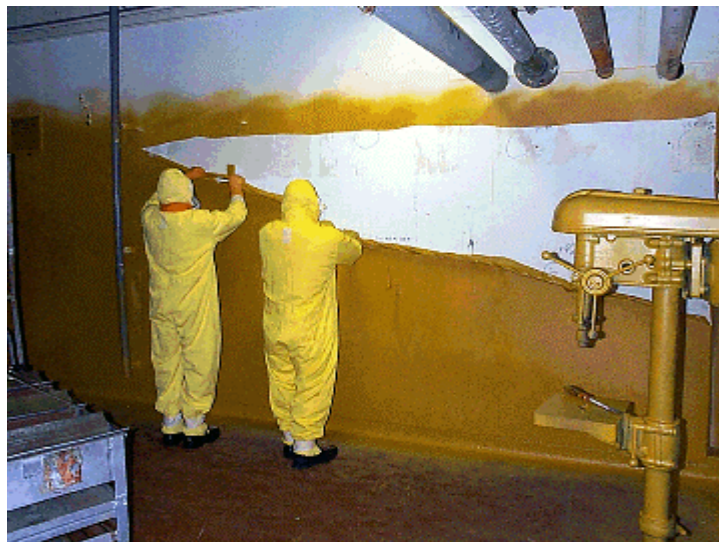
Figure 1. ALARA™ 1146 being removed from wall.
