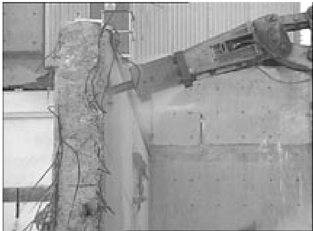
Hoe-ram with water sprays demolishing a high-wall.
