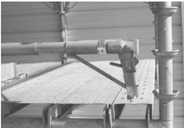
Figure 2. Excels Trigger Release Mechanism
