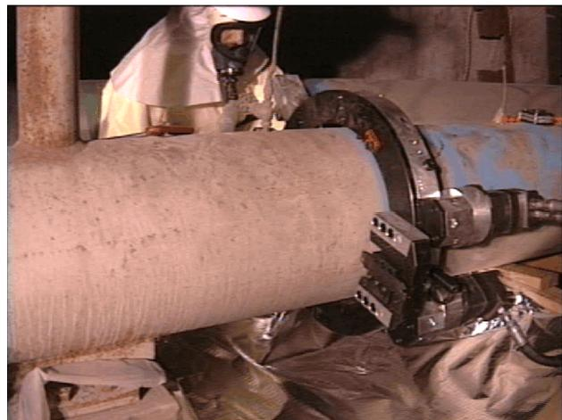
**Figure 4. Setting up to cut 41-cm (16-in.) pipe.**
