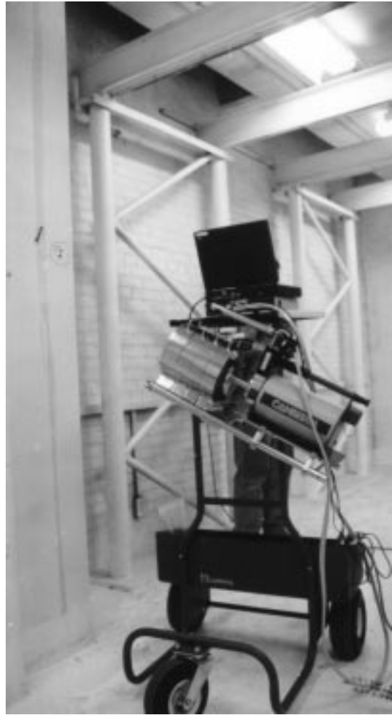
Figure 6. Survey of Hot Spot on a Wall
