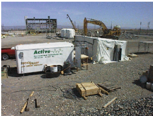
Figure 1. Decontamination trailer and pre-survey tent.
