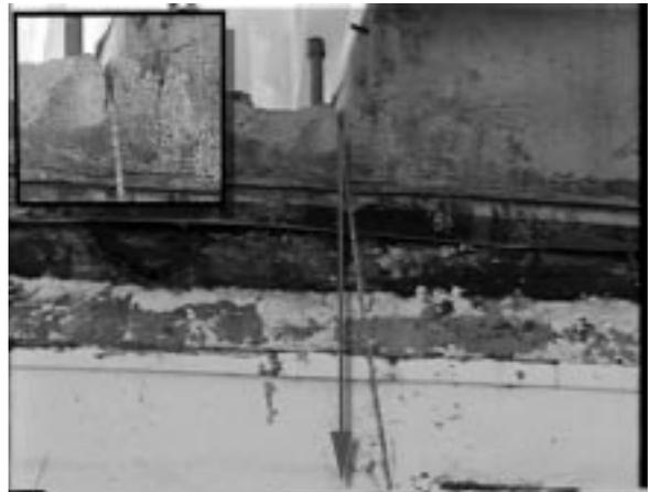
**Figure 1. Diamond wire and cut line.**
