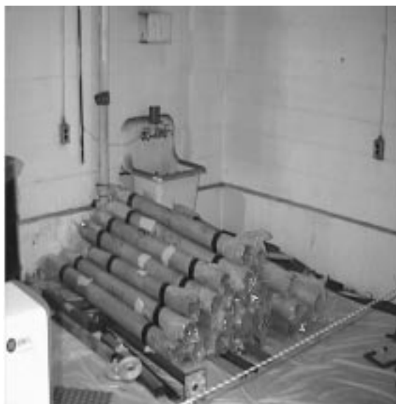
Figure 8. One lot of pipe sections monitored by the IonSens™ system.
