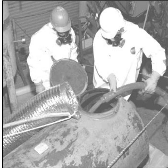
**Figure 2. Technicians inject liquid LDCC into the vessel being void filled. The vacuum hose collects fumes and airborne contamination displaced from the vessel.**
