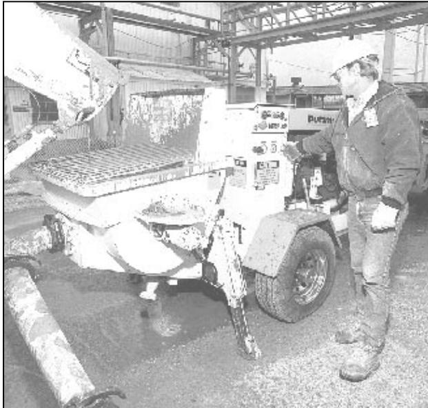
**Figure 1. The foam and concrete are combined in a concrete mixer, dispensed into a concrete hopper, and pumped to the void filling work area.**
