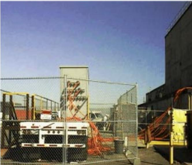
Figure 1. Portable trailer-mounted Unit Substation.
