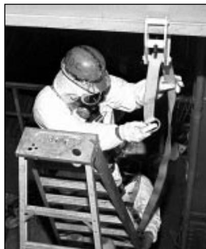
**Figure 7. Beam clamp with nylon strap.**
