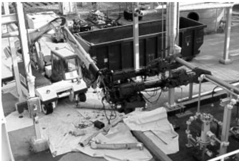
**Figure 2. Mobile Work Platform removing pipe at Fernald.**
