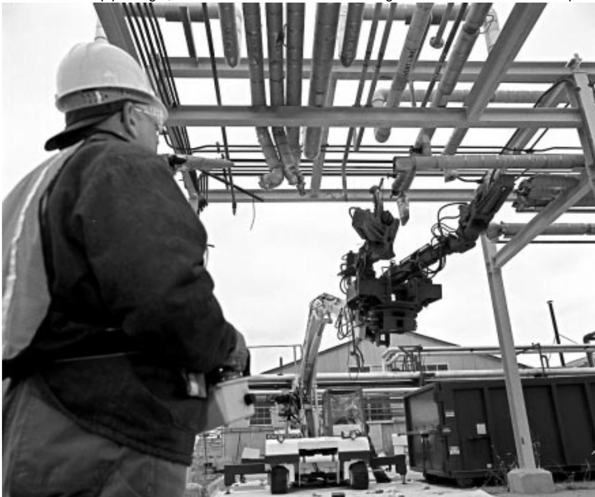
**Figure 4. MWP removing overhead pipe.**
