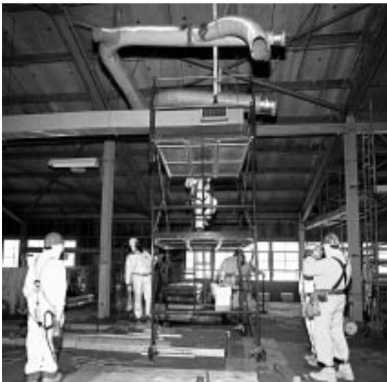
**Figure 1. Crew staging scaffolding to remove overhead pipe.**
