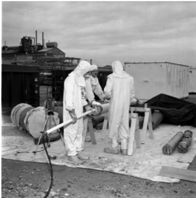
Figure 3. Workers inspecting a pipe with the BTX-II system.
