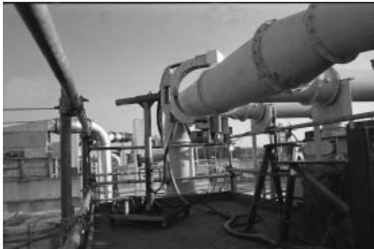
**Figure 1. Inspection Head on 20-Inch Diameter Ventilation Duct**
