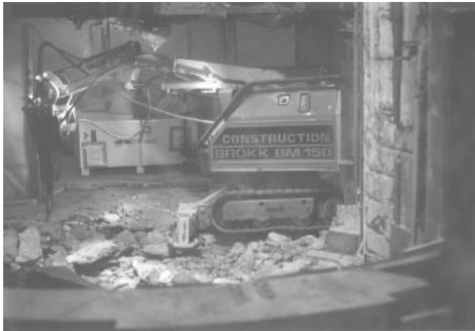
Figure 1. Brokk with hammer attachment.
