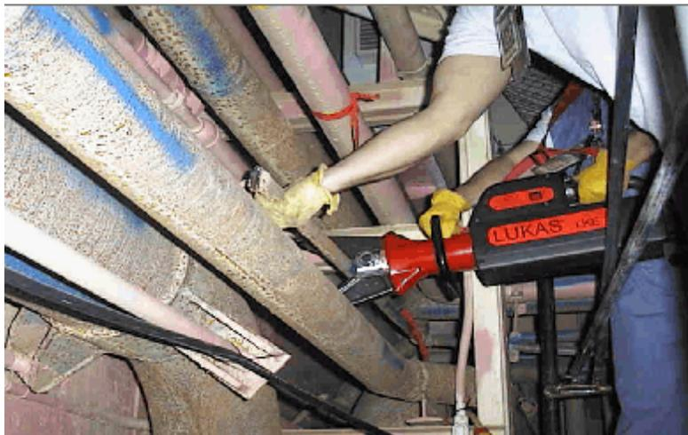
**Figure 3. Typical cutting with the innovative shear.**
