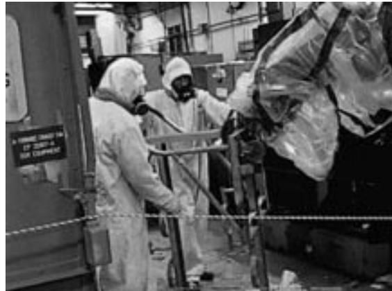
**Figure 5. Cutting Loose Items (Carts), Contaminated Area, with Head of Shear Wrapped.**
