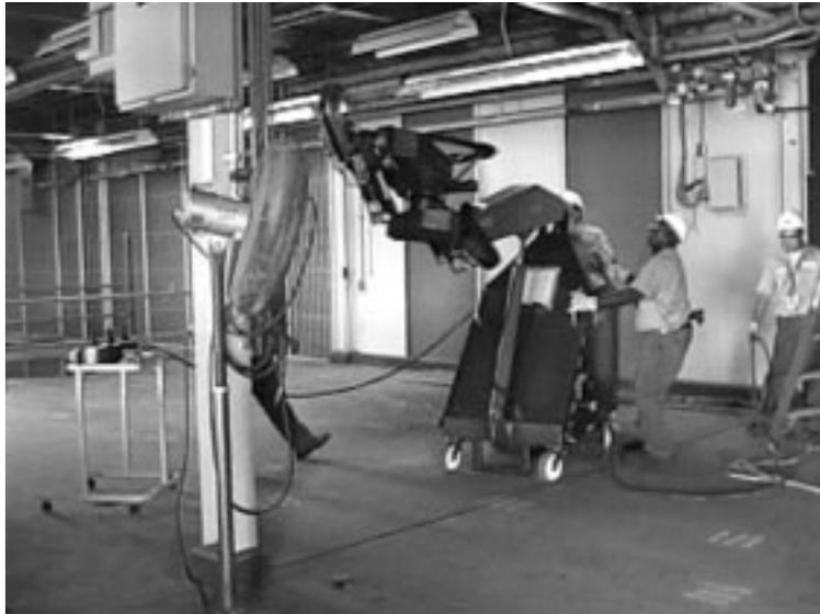
**Figure 3. Picture of SRM shear being moved into position.**
