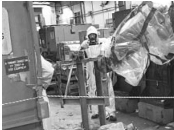
**Figure 10. Use of SRM in Airborne Radioactivity Area**
