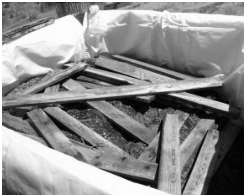
Figure 7. Loading a soft-sided container using a layered approach with soil and gravel between layers of debris.
