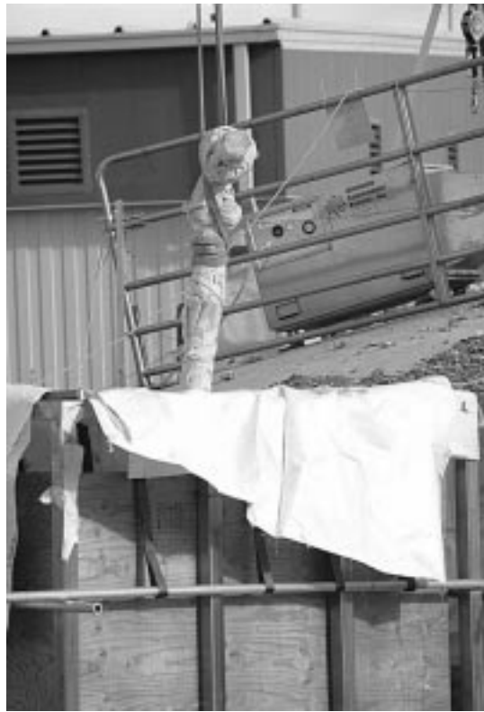
Figure 8. Removing piping from the digester and loading it in a soft-sided container.
