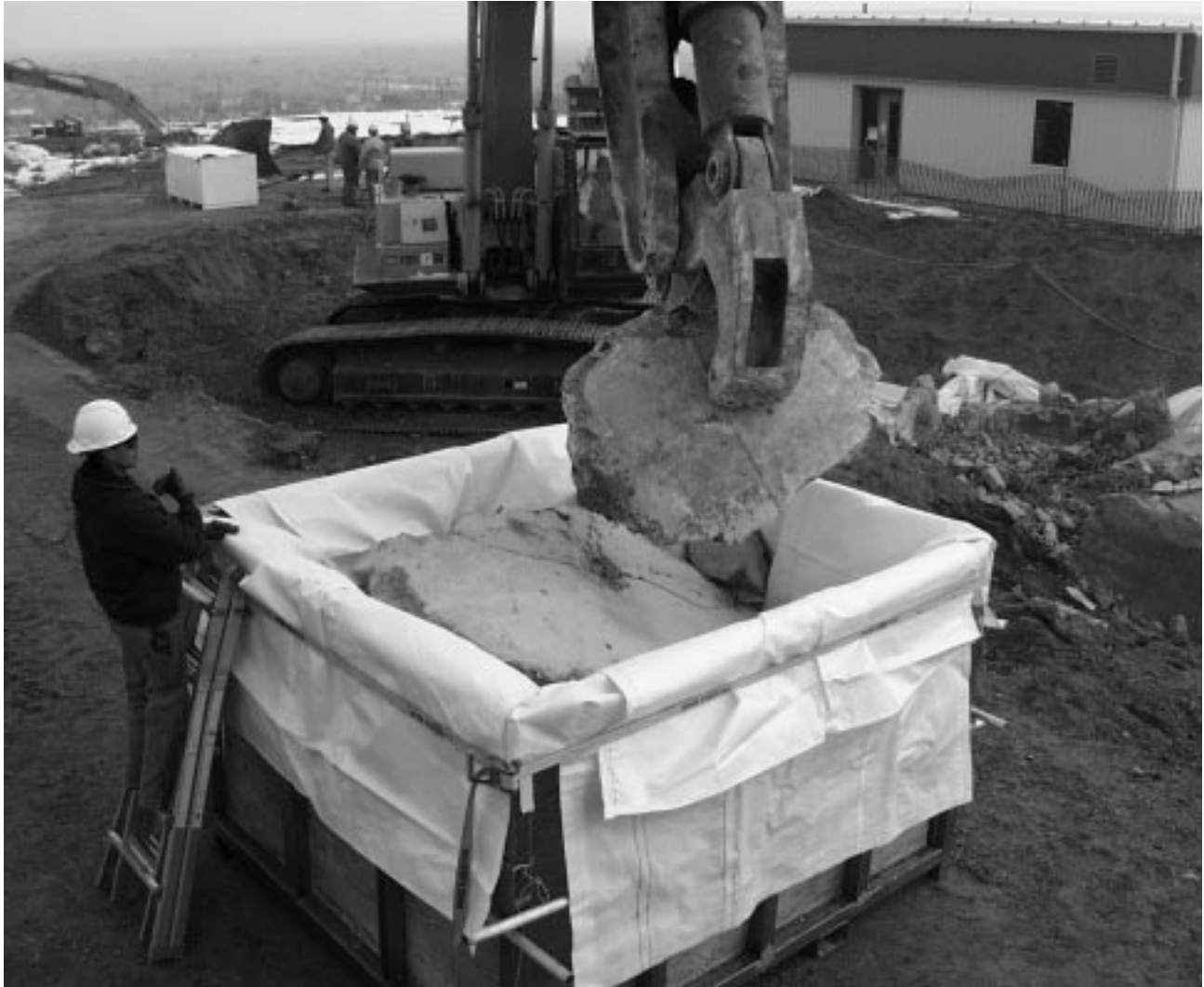
Figure 4. Filling the soft-sided waste containers with large reinforced concrete slabs.
