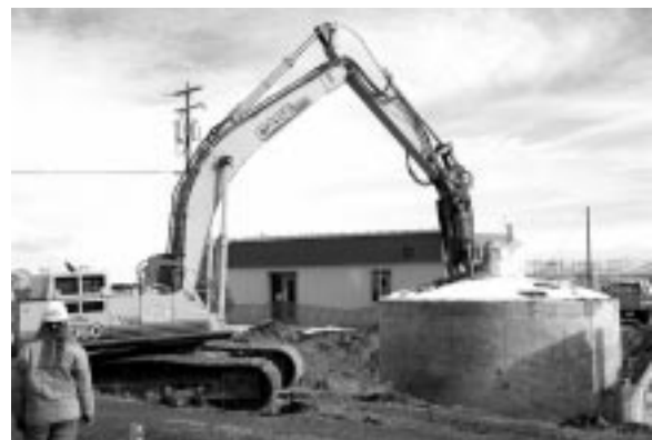
Figure 5. The Central Facilities Area Sewage Treatment Plant D&D site: digester demolition.
