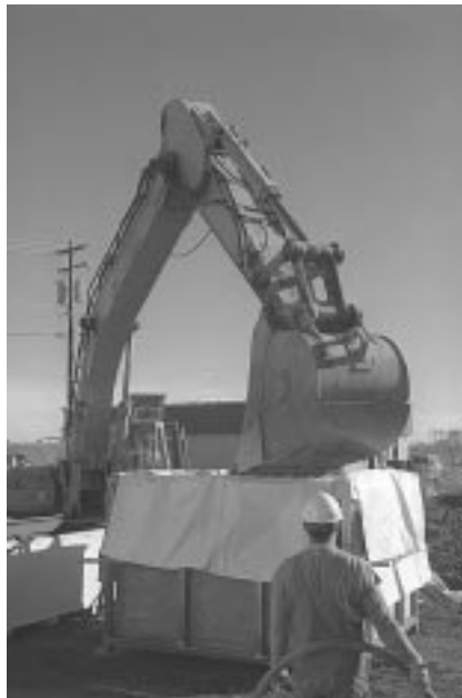
Figure 7. Loading a soft-sided container using a layered approach with soil and gravel between layers of debris.
