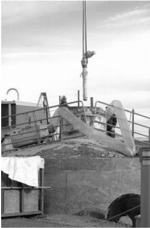
Figure 8. Removing piping from the digester and loading it in a soft-sided container.
