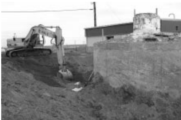
Figure 5. The Central Facilities Area Sewage Treatment Plant D&D site: digester demolition.
