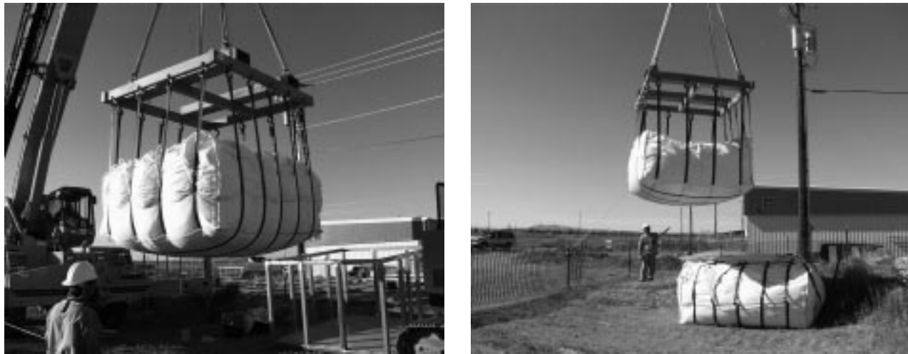
Figure 3. Lifting full soft-sided waste containers
