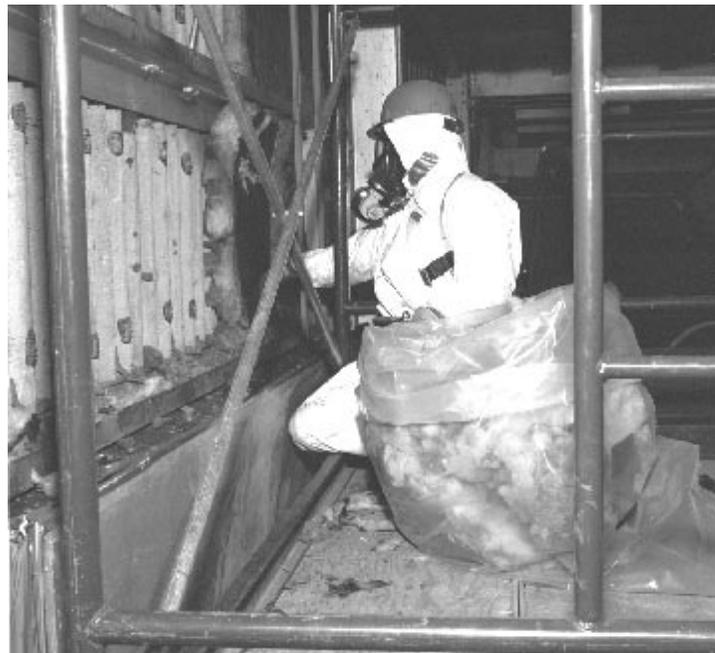
Figure 1. Worker manually removing insulation from walls.
