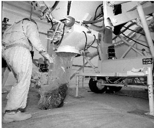
**Figure 4. Insulation removed by the VecLoader being discharged by worker into plastic bags.**
