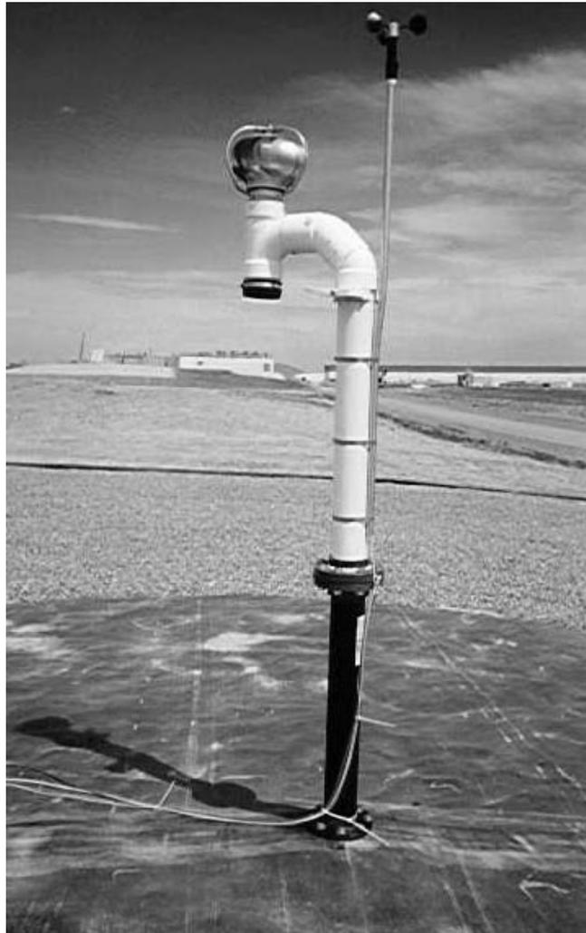
Figure 8. Photo of installed vent system over Pit 2.
