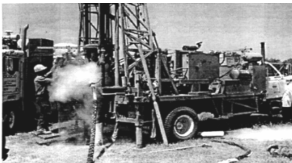
Figure 3. Cryogenic Drilling in Operation
