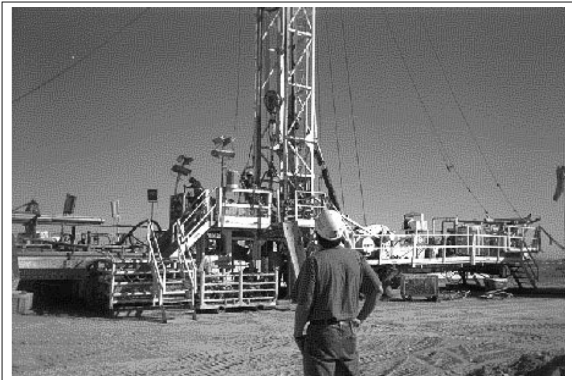
Figure 1. Conventional site surveys and site characterization are conducted using drill rigs similar to the rig pictured above. Drilling boreholes into the subsurface is expensive and adversely affects a relatively large surface area at each drill site. Contaminated material is also brought to the surface in the process, and new migration pathways may be created in the subsurface between soil and groundwater horizons.
