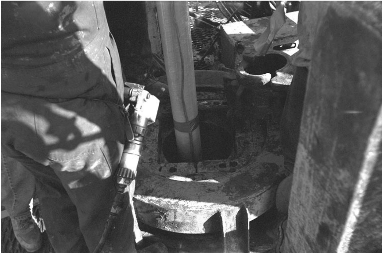
Figure 3. An electrical array with electrode dipoles attached to a supporting shaft or string is being lowered into a borehole. Once in place, the hole will be filled with grout to increase conductivity between the electrodes and the subsurface environment.
