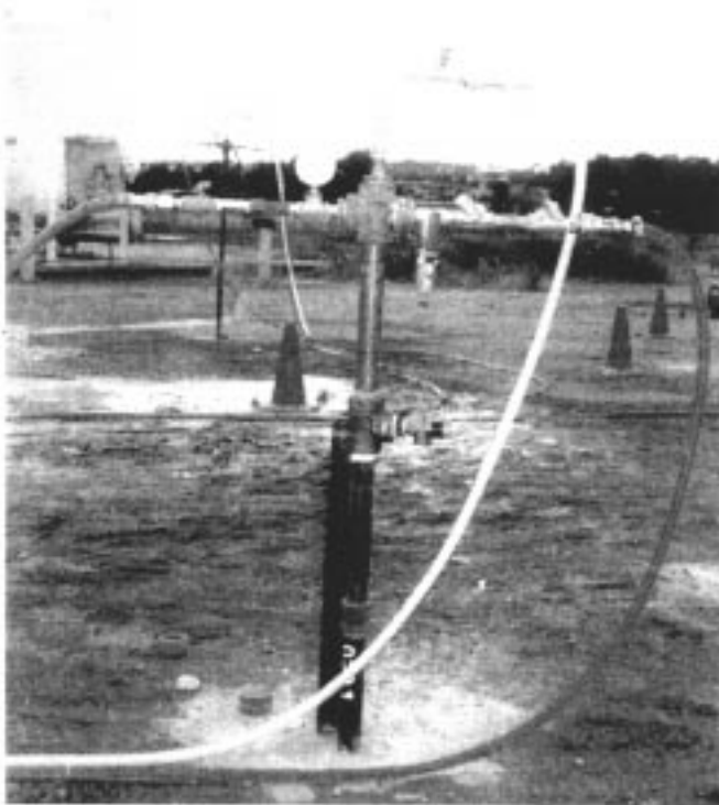
Figure 3. Photo of Geo-Cleanse® injection well.
