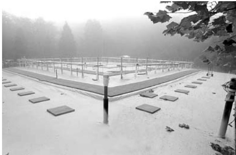
Figure 1. Frozen Soil Barrier system at Oak Ridge National Laboratory
