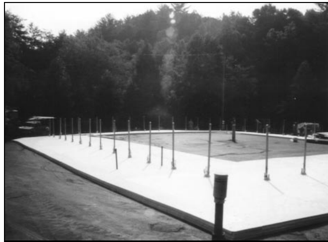
Figure 6. Insulation installed prior to membrane covering
