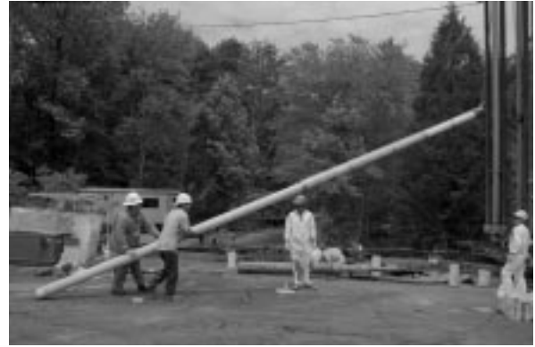
Figure 10. Thermoprobe installation
