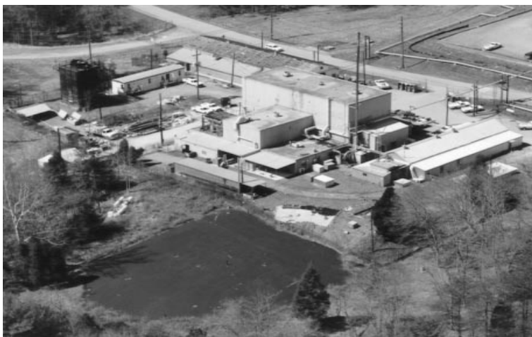
Figure 2. Demonstration area prior to installation of Frozen Soil Barrier. Impoundment is covered by asphalt cap in lower portion of photo
