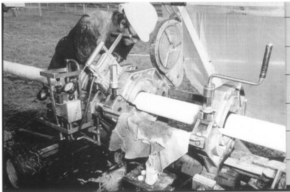
Figure 4. Assembling Schumasoil well screen at the DOE Portsmouth site.
