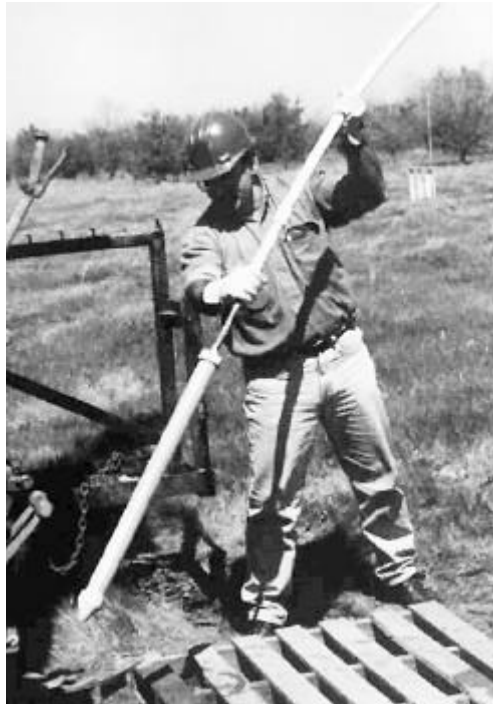
Figure 1. A flow sensor being installed through a hollow-stem auger.
