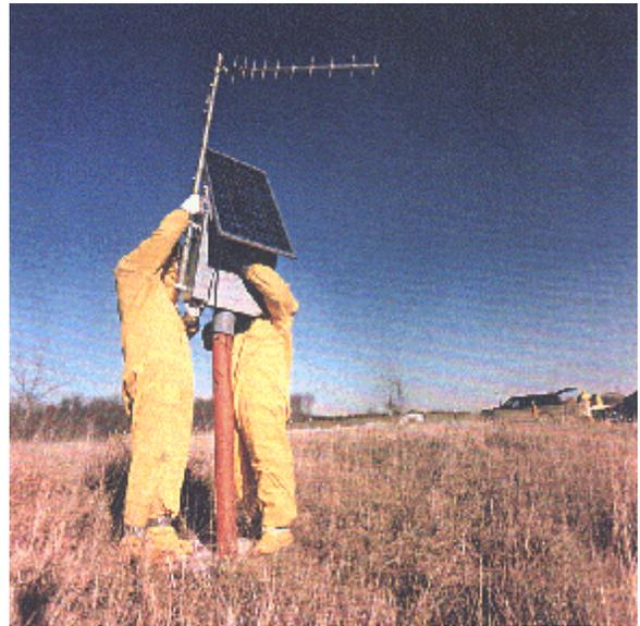
**Figure 5. Remote detector station installation on well completion pipe.**
