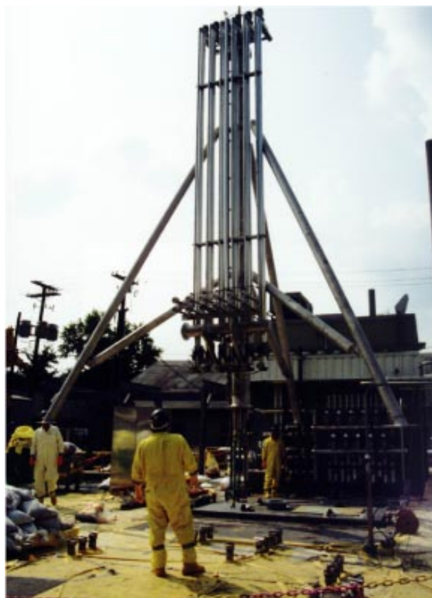
Figure 1. Installation of the jet pump skid.
