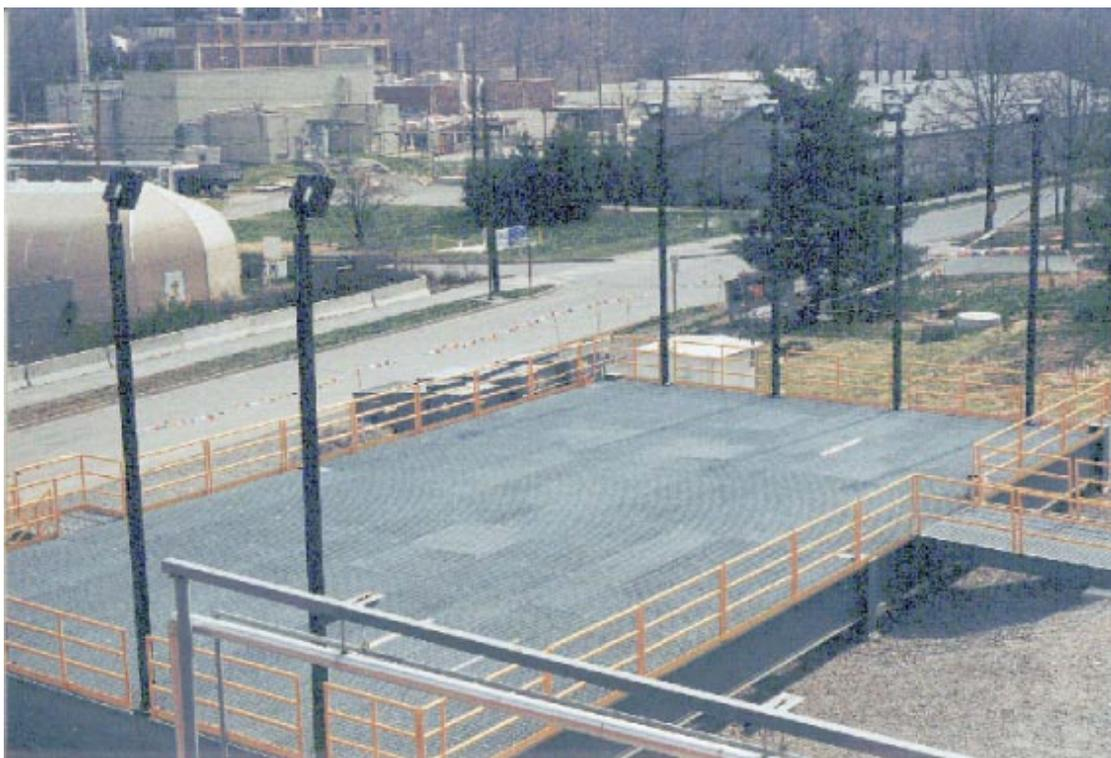
Figure 7. Load-bearing platform over Tanks W-3 and W-4.
