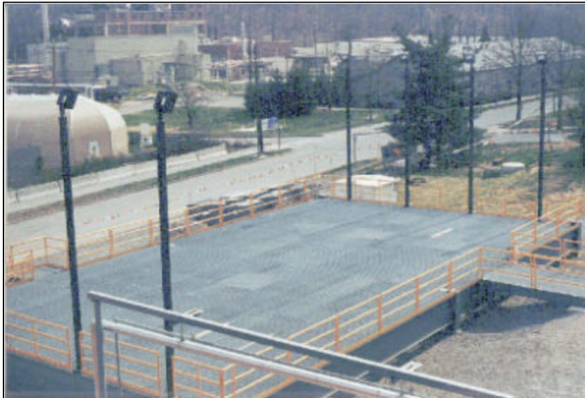
**Figure 6. Load-bearing platform bridging underground storage tanks at Oak Ridge.**
