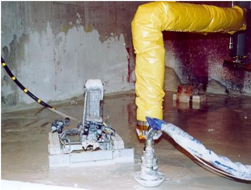
Figure 2. Modified Light Duty Utility Arm holding the Confined Sluicing End Effector and operating with Houdini and the Waste Dislodging and Conveyance System in the Cold Test Facility.
