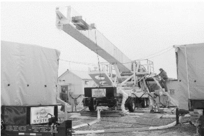
**Figure 5. Deploying the LDUA into an underground liquid radioactive waste storage tank at the INTEC tank**
