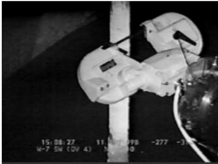
**Figure 2. Pipe Cutting Tool deployed in GAAT W-7.**
