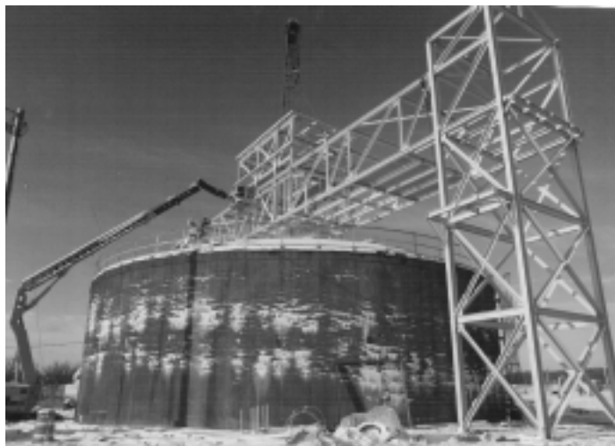
Figure 16- Silo at Fernald during construction of superstructure for Waste retrieval testing
