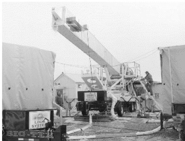
**Figure 5. Deploying the LDUA into an underground liquid radioactive waste storage tank at the INTEC tank farm.**
