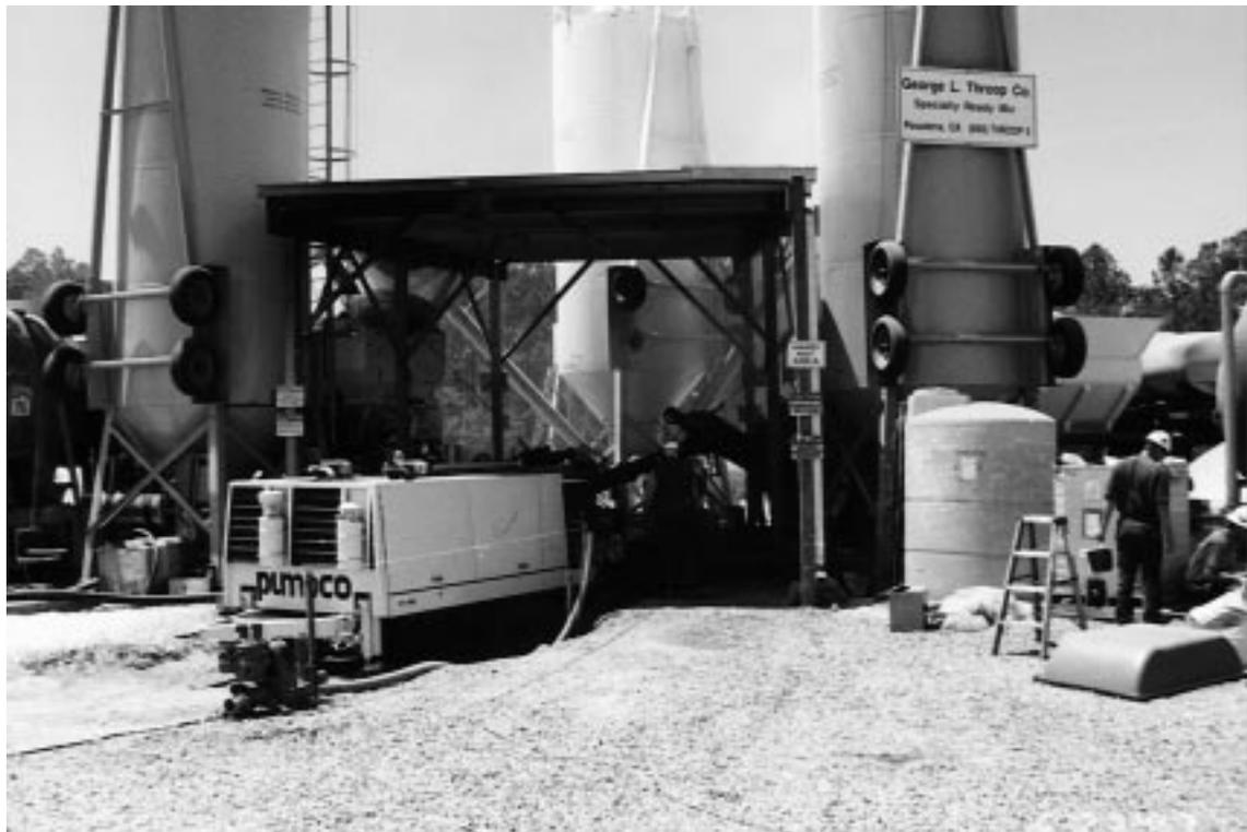
Figure 3. Grout plant used for closure of Tanks 17 and 20.
