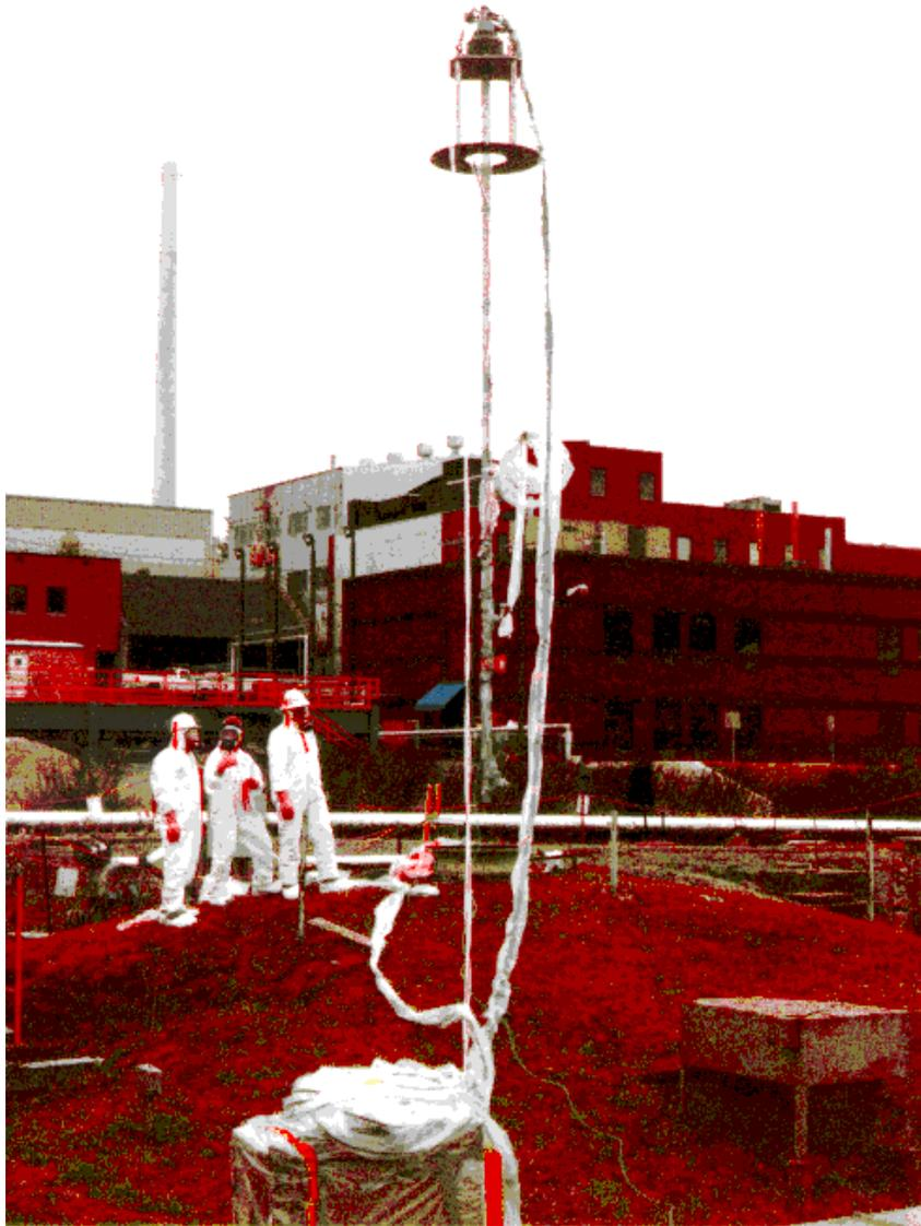
Figure B4. Topographical Mapping System installation into ORR Tank W-5.
