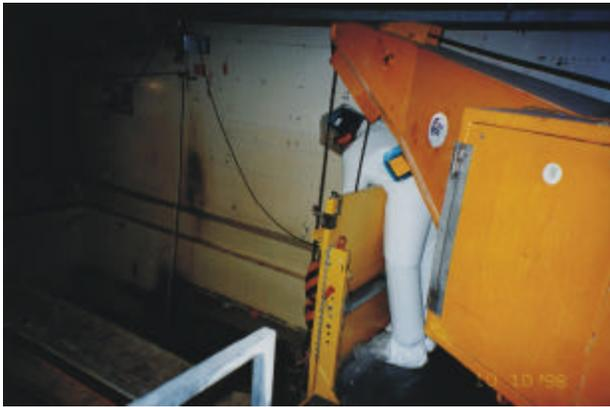
Fig. 1 Manual dismantling of the pipe duct with shielding and distance.
