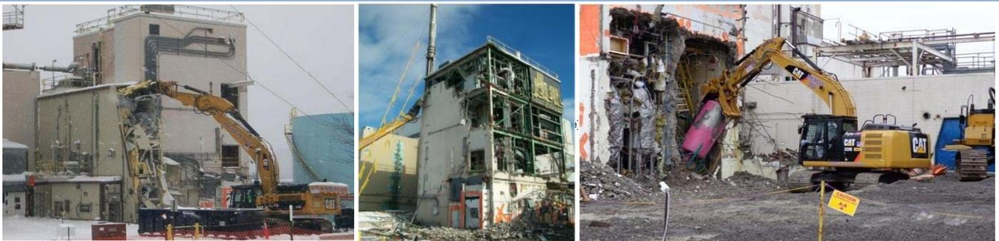
Workers demolish the West Valley Demonstration Project's largest and most complex ancillary facility, building 01-14, which was completed in July 2013. (Photos from Reference 2)
