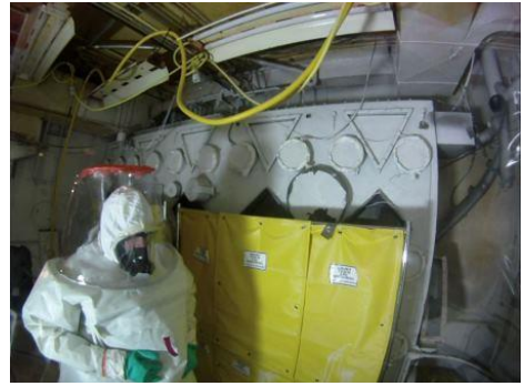
A CH2M HILL employee wore specialized respiratory equipment and protective suits when entering one of the most hazardous rooms at the Hanford Site in September 2014, increasing protection from high radiation levels and heat stress.
